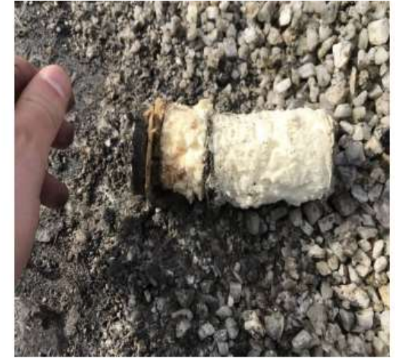
Picture of roofing system layers: Asphalt Membrane/reinforced felts, coverboard, tapered insulation & vapor barrier.
